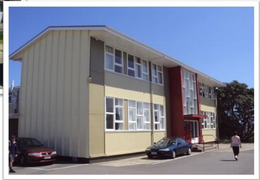
Half Nelson two storey (“T” block)
